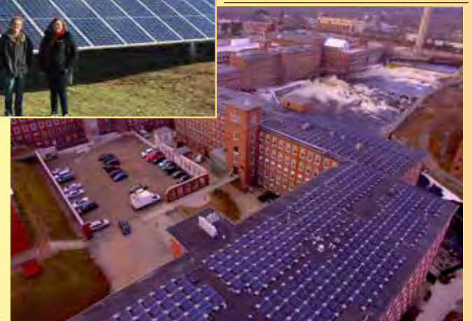
Below: Pepperell Mills in Biddeford, Maine. It is Maine's largest privately-owned solar array consisting of 1,192 panels over 1.5 acres of rooftop and producing 437,320 kilowatt hours of electricity annually.
