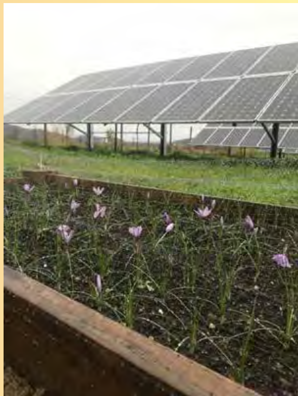
Saffron crocuses blooming in a raised bed within a Peck Solar array in New Haven, VT. Image: A. Ghalehgalabbehbahani, UVM.
