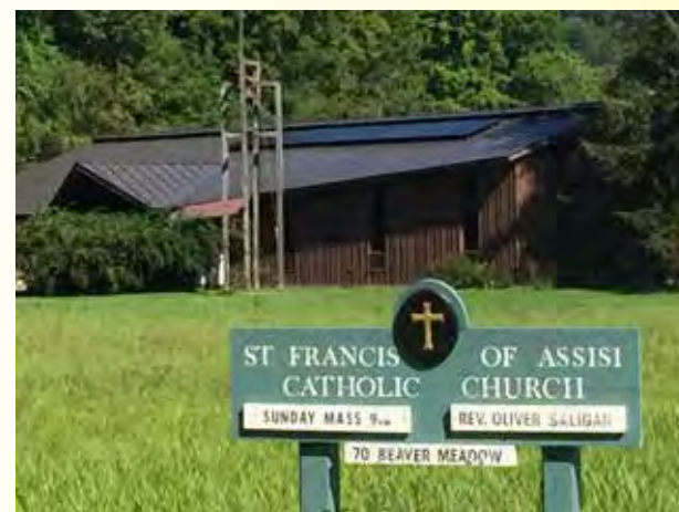
The St. Francis of Assisi rooftop solar array has twelve solar panels, for a capacity of 3.96kW.
