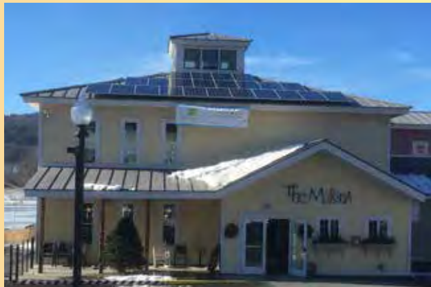
Integrated Solar Applications installed this east-west and south solar array on The Marina restaurant in Brattleboro, VT. Photo: Integrated Solar Applications.
