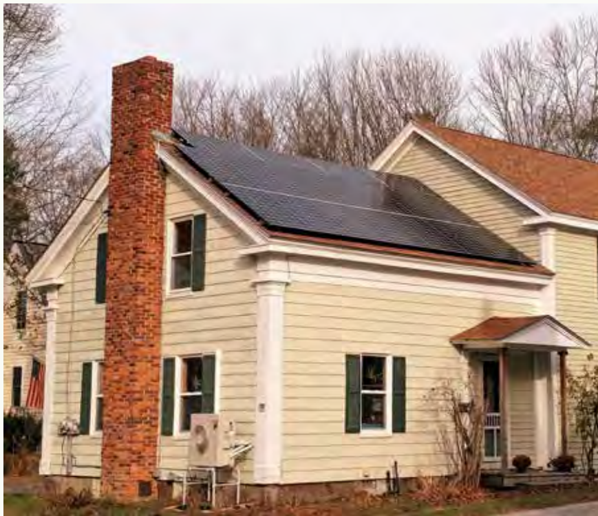
A 6.3kW grid-tied solar electric system paired with two single zone Mitsubishi heat pumps in Bath, Maine. Image: Maine Solar Solutions.
