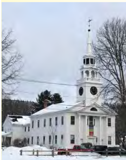
Norwich Solar Technology's EZ-PV MetaModule™ system in action at the Norwich Congregational Church. All photos courtesy of Norwich Solar Technologies.
