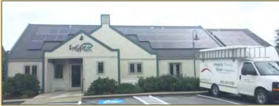
Integrity Energy, LLC installed the solar system on the east and west-facing roofs to provide 100% of the energy needed for the EyeCare For You office in Bethel, VT. Photo: NR Mallery.
