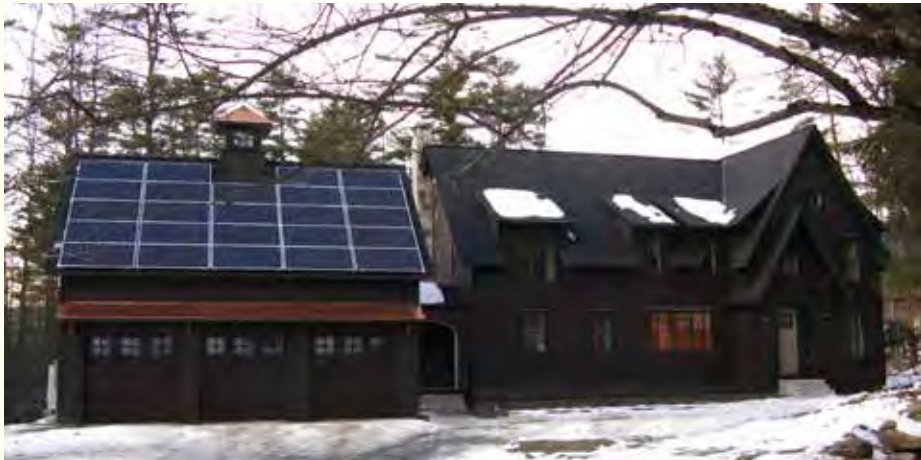
The Kaiser Gish house in Hanover, NH is retrofitted to achieve net-zero status. It includes three all-weather air-source heat pumps and an 8-kW rooftop solar array. Photos by Karl Kemnitzer.
