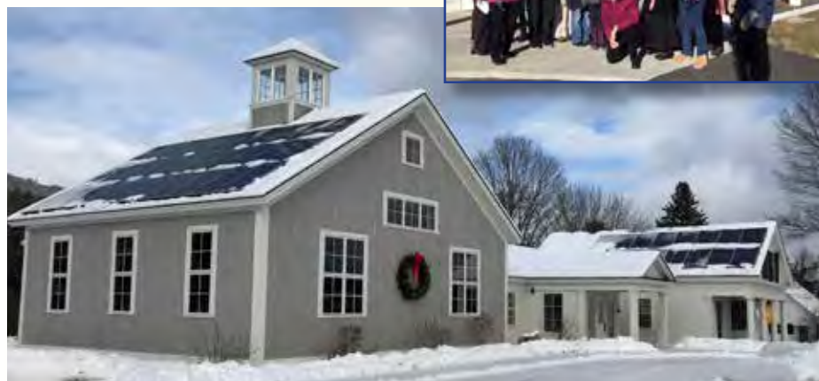
The Unitarian Universalist Church of the Upper Valley has a rooftop array consisting of 45 panels providing a total power of 15.75kW DC.
